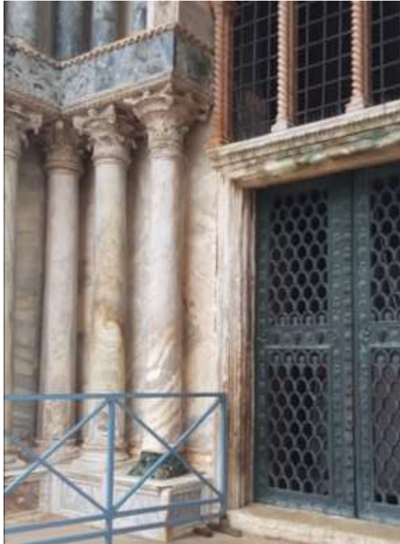
Figure 10. The effects of increased pressure by salty water, air pollution (SOx), and more intense use on the basis of two marbles columns of the St Mark's Basilica front
