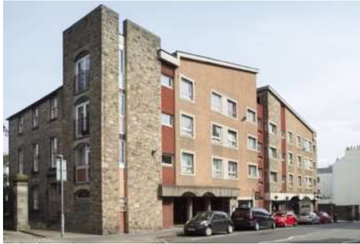
Figure 7. EWH promoted a project to improve energy efficiency of this 1969 building
